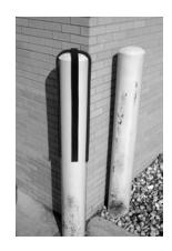
2. Slide the Post Guard over the bollard.
